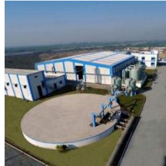
Tertiary Wastewater treatment plant
