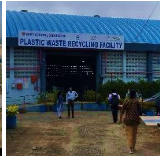
Plastic Waste Recycle Facility
